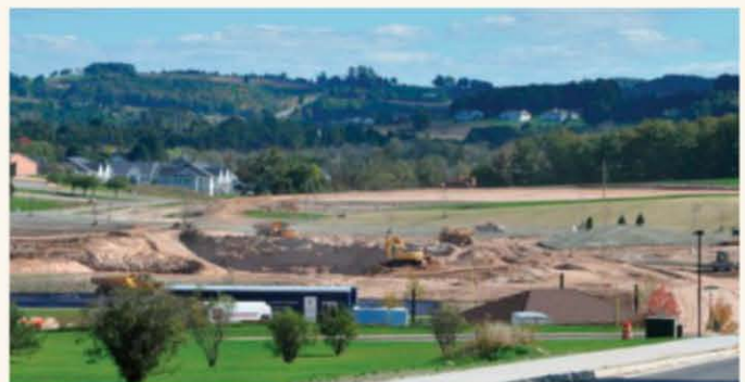
BIG CHANGES UNDERWAY AT THE PETOSKEY SCHOOLS' CAMPUS.
